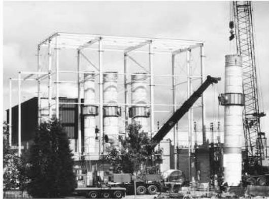
Fig. 12a. Multiple effect vertical tube evaporators (courtesy of APV Crepac Inc.)
